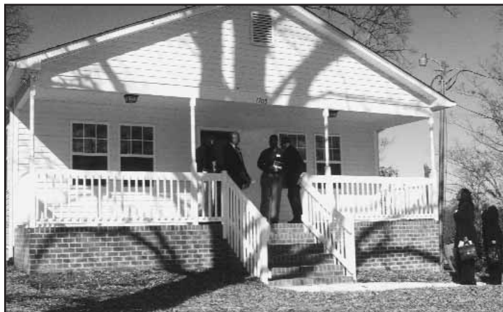
Following lunch and the dedication service, guests were invited to tour the new homes. In addition to the bedrooms, the homes have three baths, washer/dryer space, kitchen and living areas.
