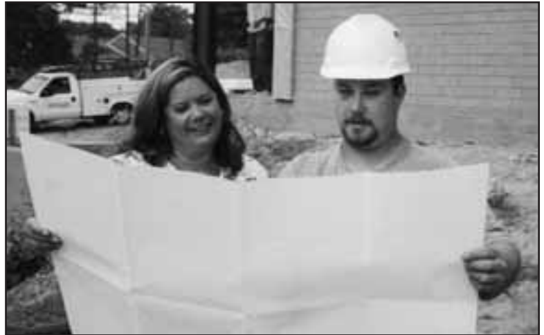
Jon Gilland shows Stacy Jesso where DuctSox (Fabric Duct System) technology is being incorporated into a portion of the HVAC system in the new Kennedy Campus sports and activities center. DuctSox provides an economical and aesthetic HVAC air distribution system.
