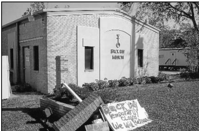
Elon Homes will be sending a work crew to assist with rebuilding efforts in the severely impacted area.
